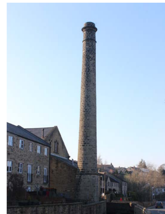
Grade II Listed Mill Chimney
