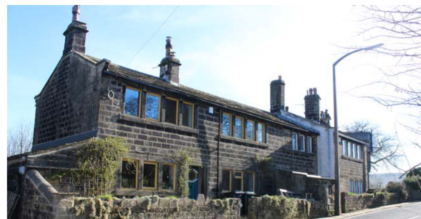
13 & 17 Hebden Bridge Road
